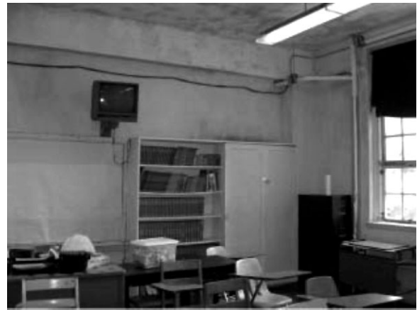
FIGURE 2. Picture of classroom wall and ceiling showing active mold growth at the water-damaged school.
